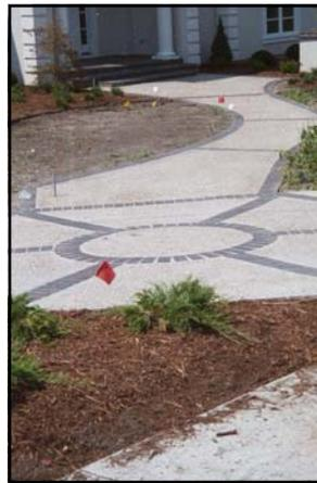
This means, in addition to transverse jointing, a joint must be cut down the center for the full length of a driveway that is 12 feet wide and 4 inches thick, or for one that is 16 feet wide and 6 inches thick. Joints usually are at much shorter intervals in public sidewalks. Most common spacing is 5 feet. Local codes or ordinances govern. Joints must be straight and continuous, not staggered or offset.
